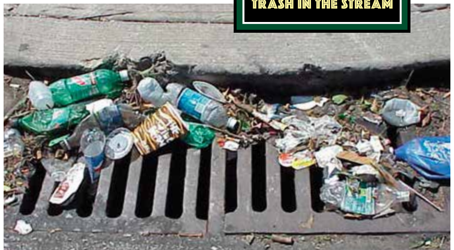
Trash accumulates and clogs a storm drain. Some of this trash will end up in our local waterways.
