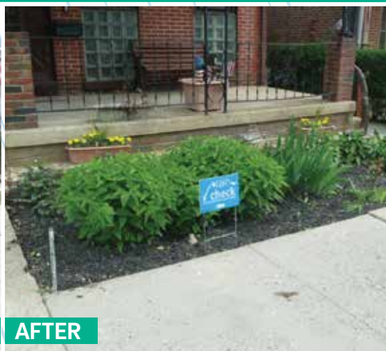
DE-PAVING BY INSTALLING A RAIN GARDEN
